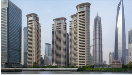
Tomson Riviera Apartment Towers Shanghai, China
